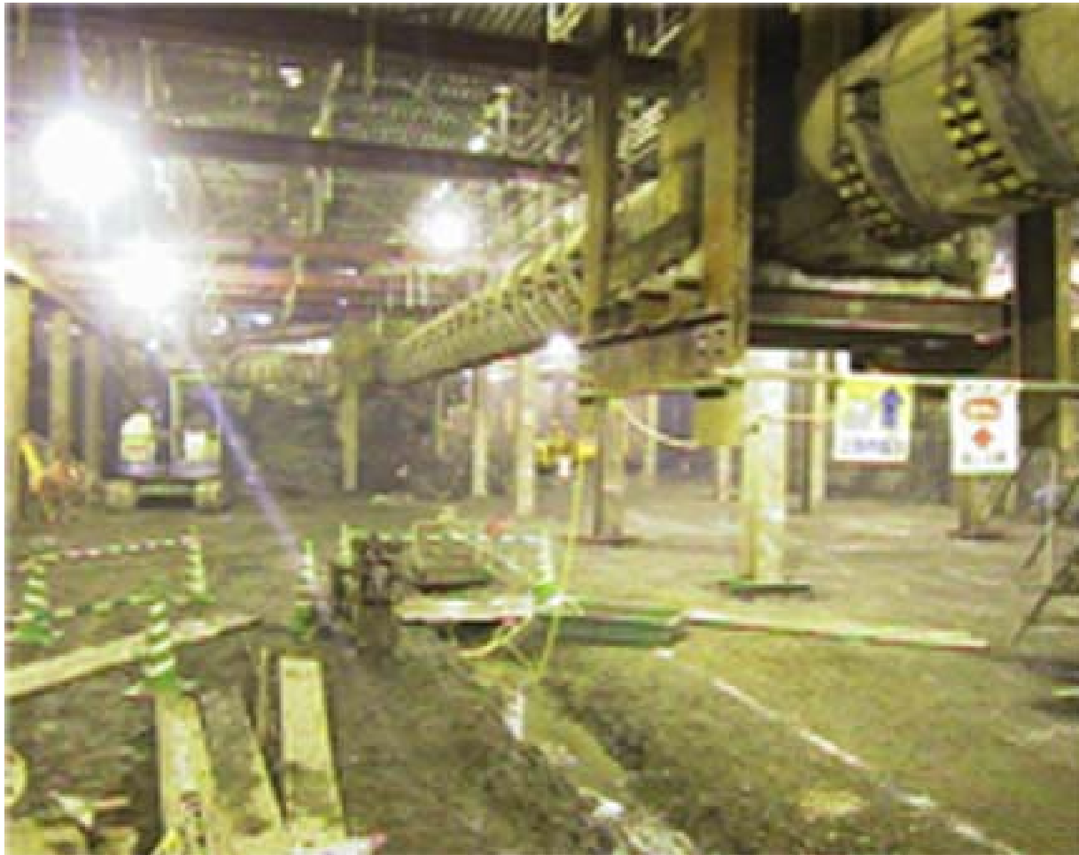
Fig. 2.6. The situation of construction
